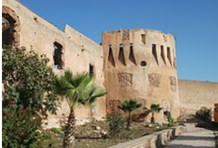
Azemmour (fascinating wall conception by Francisco de Arruda who reinforced the former city walls with an ancestor of Renaissance bastions.)
